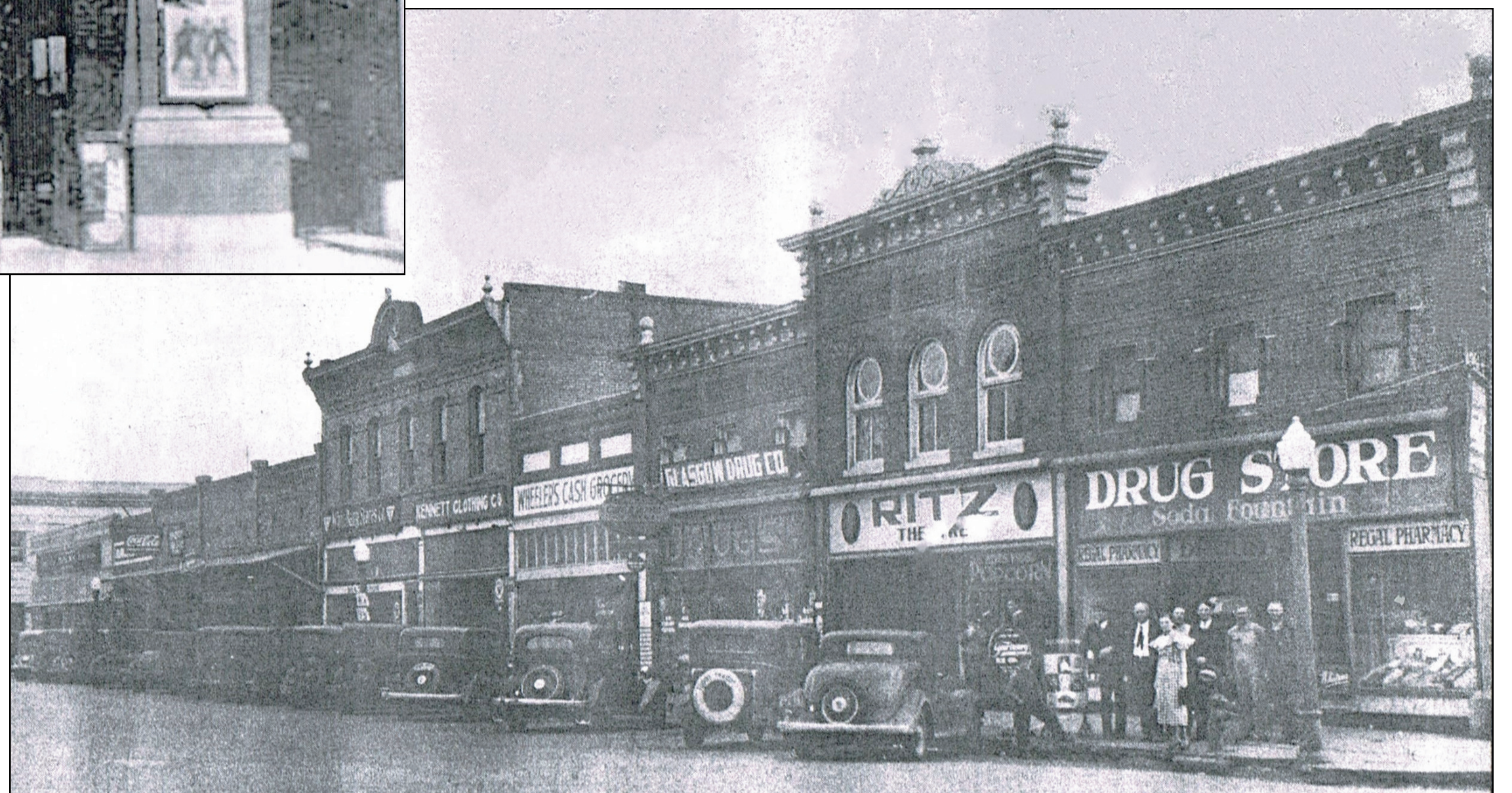
The Ritz Theater (second building from right) on the South side of the square, 1933.
